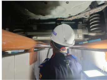
Gambar 40. Sistem manajemen residual energy storage system (ress)
